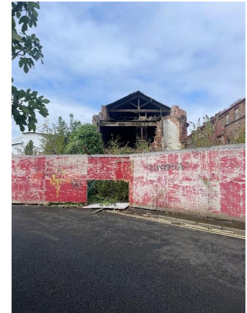
Figure 35: The east end of the building has totally collapsed, opening the east elevation up and allowing water to penetrate the structures, causing decay.
